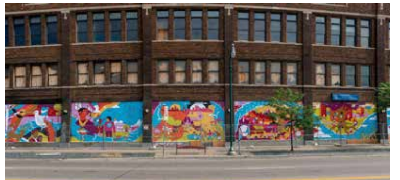
The Coliseum building renovation nearing completion
