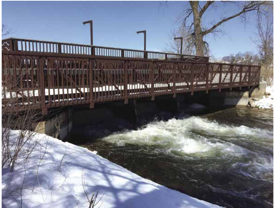
Gray's Bay Dam
